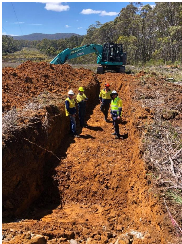
Figure 1 Test pitting
